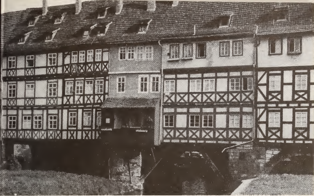
The Krämer Bridge in Erfurt, built in 1325
